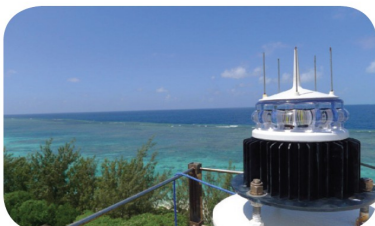
Jomard Island, Milne Bay, Papua New Guinea Image supplied by Nawae Construction
